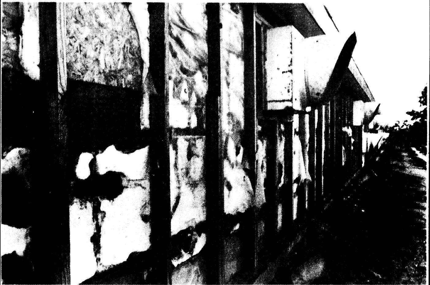
Figure 1 Rats penetrated the walls of this swine finishing barn, completely destroying the insulation. It had been reinsulated only 2 years previously (Photo courtesy of National Hog Farmer magazine).
