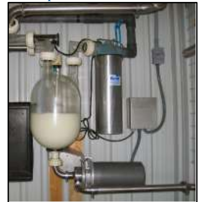
Fig. 8 Receiver jar with milk pump and trap
